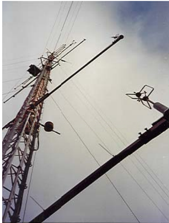
Fig. 1.5. Micro-meteorological tower experiment at Sodankylä. The mast with a height of 48 m is installed into a Scots pine forests on sandy soil measuring eddy-covariance fluxes of \text{CO}_2 , latent and sensible heat and momentum, radiation components, and gradients of the \text{CO}_2 concentration, temperature and wind. Soil, vegetation and snow parameters are also monitored in the forest region around the tower.
