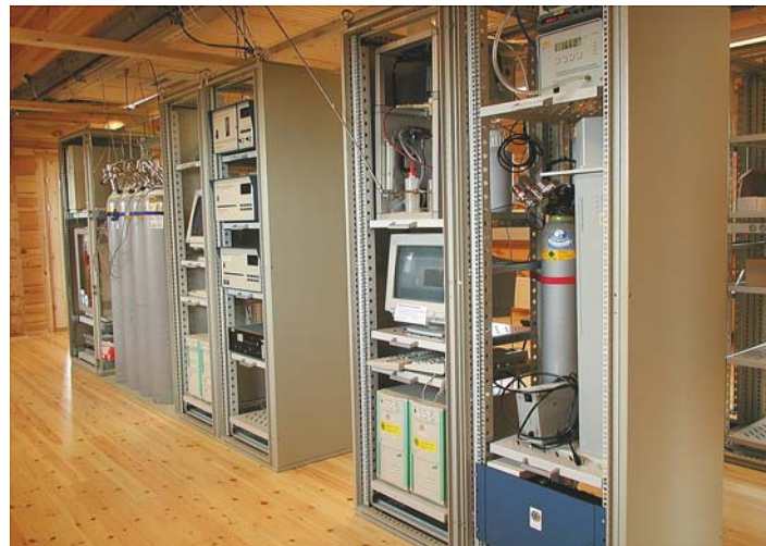
Fig. 1.9. The Sammaltunturi station at the Pallas site.
