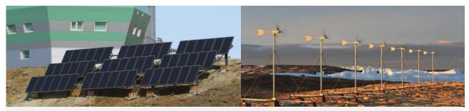
10 kW Solar PVs (left) and 21kW Wind Power Plants (right) in Operation at Zhong Shan Station (Photo: PRIC)
